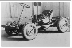
Above: Chassis of the 2<sup>nd</sup> WAC prototype showing the frame and position of the air-cooled mid-engine. (Photo: US Army)
