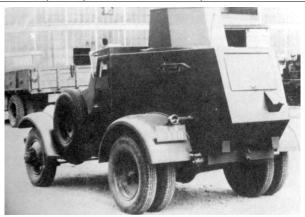
Remarks: Designed by US Army Quartermaster Corps, with Franklin air-cooled engine, 4x4, circa 1931. The third version of the T6 was actually modified from a T7 Armored Car. The Quartermaster developed T6 had the same general layout and characteristics as the T7 except
