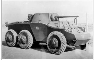
Above: The Studebaker T21 had a non-powered front axle so was actually a 6x4 vehicle. (Photo: US Army)
