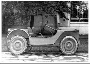
Above: The single Ford extra light 1/4-ton completed. Ford ended up withholding the vehicle from testing. (Photo: US Army) **Remarks**: Although designed for the extra lightweight 1/4-ton requirement, the Ford vehicle wasn't submitted for evaluation. Only the single prototype was completed. Fitted with a Ford tractor engine, the little vehicle would have been badly under powered.
