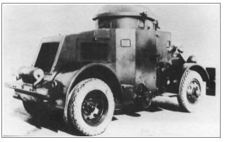
Remarks: Ordnance design built by FWD/Marmon-Herrington, 4x4, circa 1932. The pilot T11 was tested at Aberdeen Proving Ground from January to July of 1933. As delivered by FWD, the car had several problems including mechanical failures due to insufficient strength of the rear end. Despite the problems, an order for six cars was issued which the Marmon-Herrington Company would complete, building five T11E1s and a single T11E2. Vehicle Data: Weight Empty, 9,750 lbs (4427 kgs).
