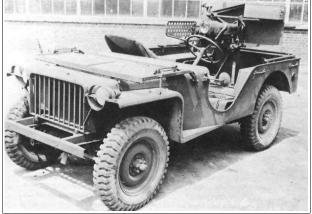
Above: Carr, Wpns, 4x4, Carriage, Motor, 37mm Gun, T2. Remarks: Based on the "Bantam" 1/4-ton Truck, Reconnaissance. A 37mm anti-tank gun with shield was moun-
