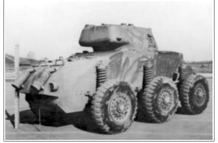
**Remarks**: Chevrolet, 6x6. low silhouette, developed into T28 Armored Car. Two pilot models built, one as T19 and one as T19E1. Armament one 37mm cannon and two .30 caliber LMGs. Armor .25 to .5 inches. Weight 28,500 lb., max. Speed 55 mph. circa 1942. The Armored Car, T19, was a 6x6 car with independently sprung wheels and an attempt to provide improved rideablility over the then current 4x4 and 6x6 designs. Construction of two pi-
