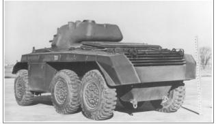
**Remarks**: The Ford, "Deerhound", 6x4, had a limited production run of 250 cars and was used internally in the U.S. during WWII. The Armored Car, T17, carried a crew of four and weighed in at 28,390 pounds (2,079kgs) unloaded. The frontal armor was from 1.25 to 2 inches
