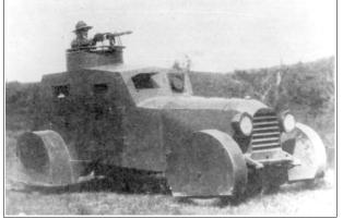
**Remarks**: An independent project, the 112<sup>th</sup> Cavalry vehicle was designed and built by Cpt. John B. Dunlap. *Armament:* (1) .30 cal. machine gun. Elevation, manual. Traverse, 360 degrees. Crew, 3-4. *Engine:* Type, gasoline. Location, forward. Cooling, liquid. *Transmission:* Type, manual. *Suspension System:* Type, leaf spring. Steering, front axle. No of wheels, 4. *Performance:* Speed/Land, 70 mph (112 km/h). Drive, 4x2. *Usage:* US Army, trial vehicle only.
