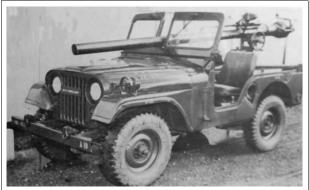
Above: M38A1C with Rifle: 106mm, M40A1 with Mount Rifle: 106mm M79. This combination was to become the standard for the M38A1C. (Photo: US Army)
