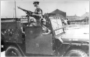
Above: Typical of the field improvised armor fittings used on the 1/4-tons, this conversion used salvaged armor plate and ingenuity, along with almost no protection from the front. (Photo: US Army)
