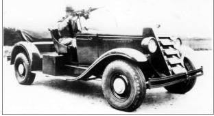
Remarks: The T3 was a refined version of the T1 Armored Car and the T1 Cavalry Scout Car. Basically the rear seats were changed from two separate seats to a single bench; and radiator armor was added along with the armor plate in front of the driver and gunner. Additional changes included a 15-volt electrical system for the radio equipment, strengthening the front axle and installing a machine gun mount.
